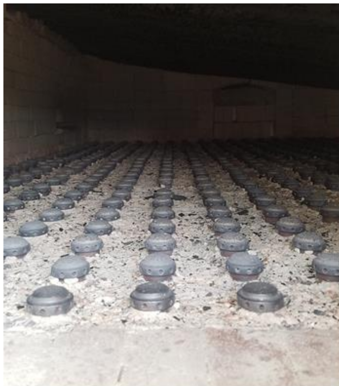
Figure 2: Combustion chamber of fluidized bed boiler
