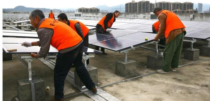
Typically, factories will install the solar system on available and suitable **rooftop** space, but you can also install the system if you have available space **near the factory** (ground-mounted).
