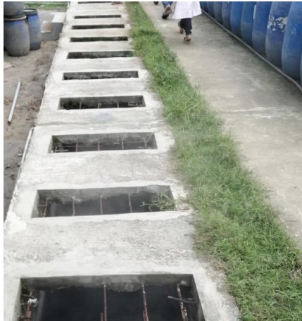
Effluent channels
