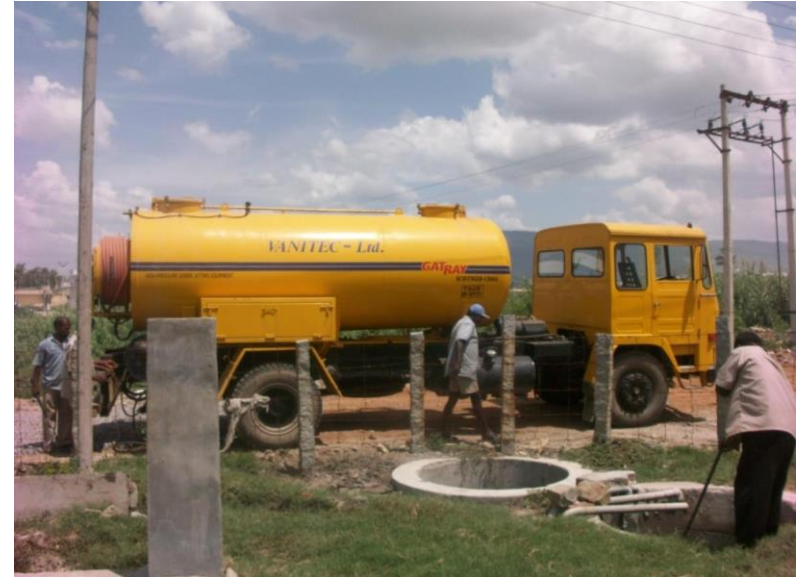
Mechanical cleaning at VANITEC CETP
