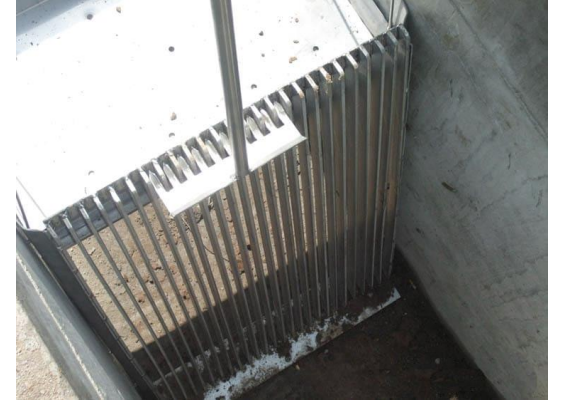
Rake and spindle for cleaning screen
