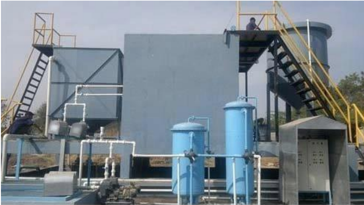
Fenton treatment unit by Xh2o Solutions Pvt. Ltd
