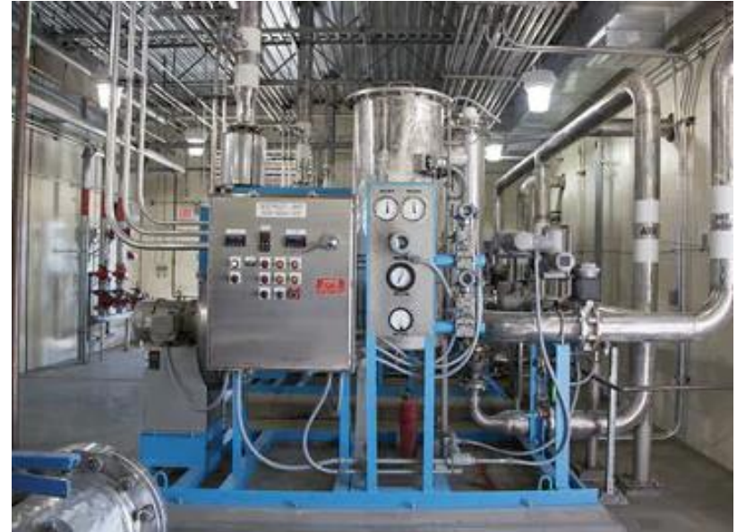
Ozonator (at Wylie Water Treatment Plant, North Texas)
