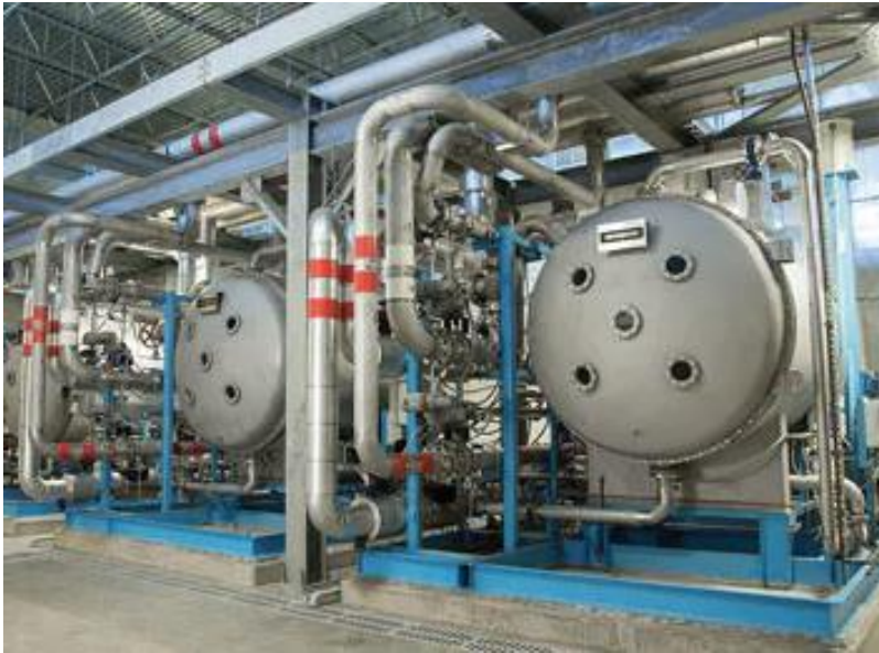
Ozonator (at Wylie Water Treatment Plant, North Texas)
