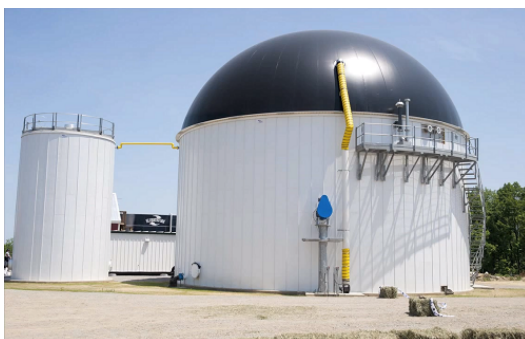
Figure 4 A sludge digester in Massachusetts, USA 3
