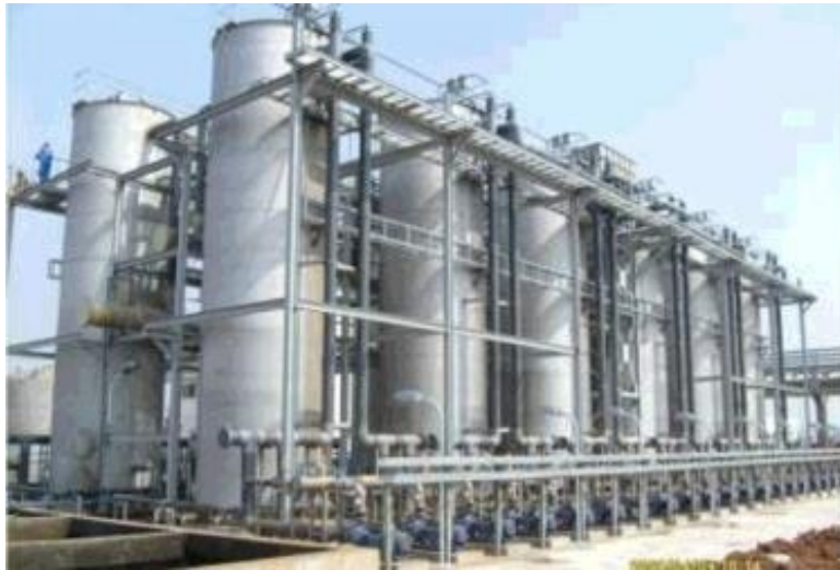
Fluidized Fenton reactor (Source: Science Direct)
