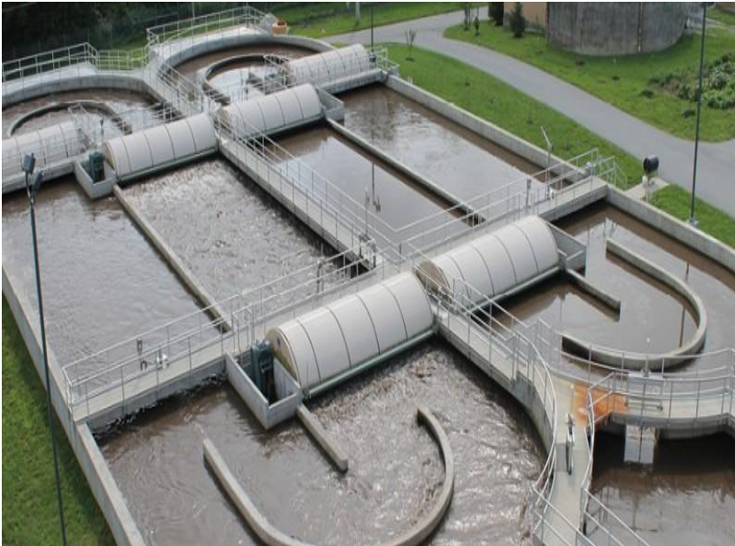
Image: Lakeside equipment
