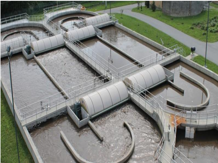
Image: Lakeside equipment
