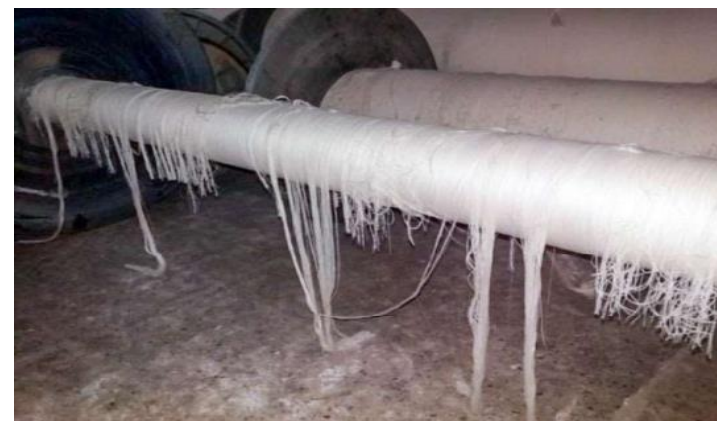
Residual beam wastage
