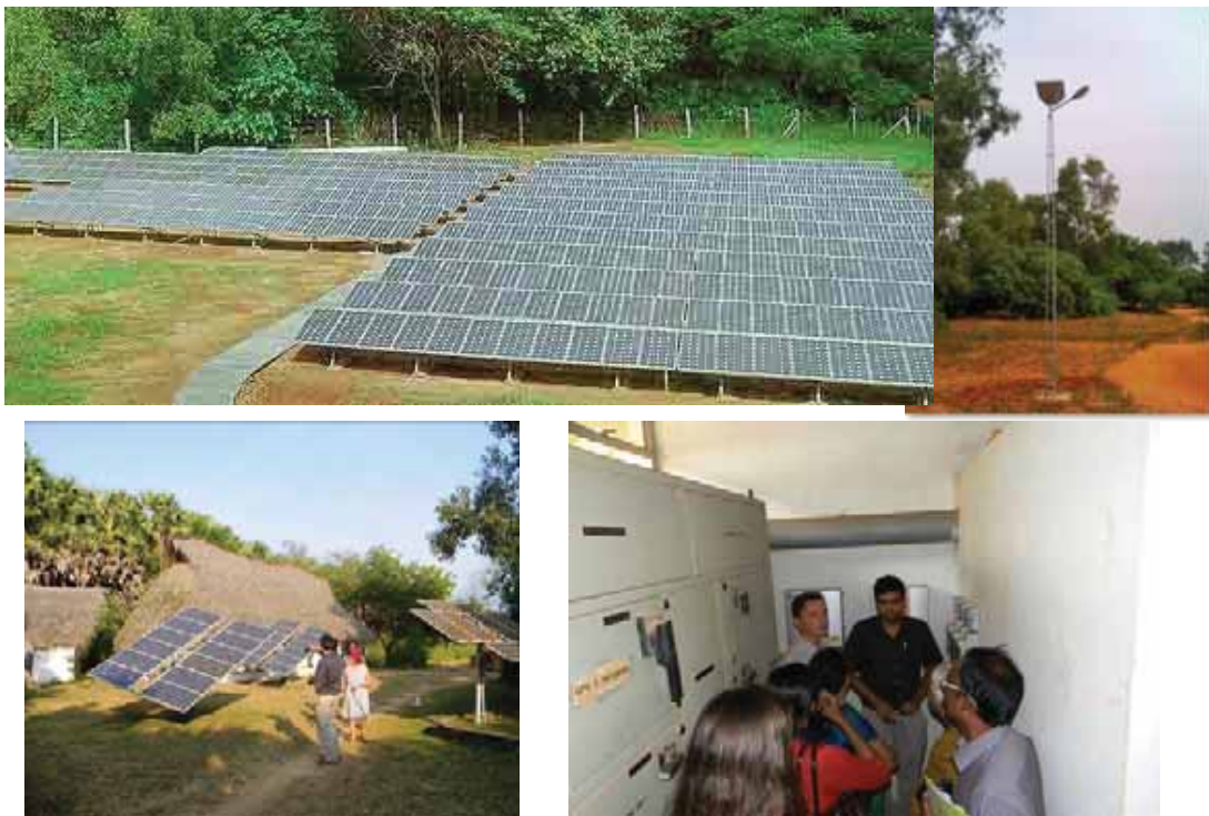
Pic. 3.10: Visit to Photo Voltaic Installations at Auroville
