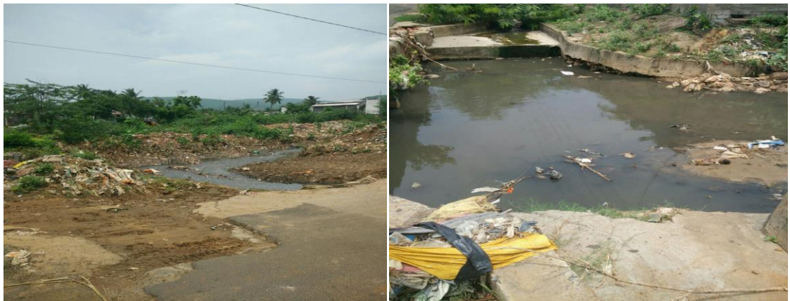
Figure 5: Garbage Disposal impacts on Drainage System
