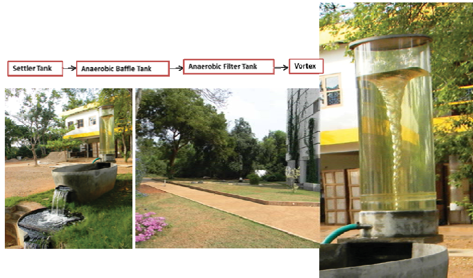
Image no. 3-31: Decentralized treatment system with Schauberger vortices
