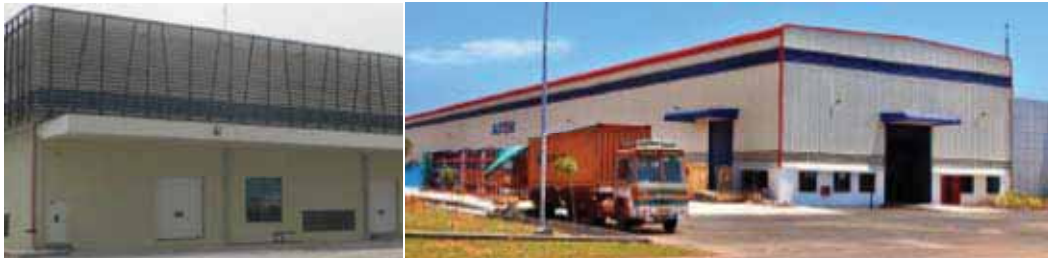
Image no. 3-20: Examples of Green Factory Buildings at Sri City, Tada, Andhra Pradesh
