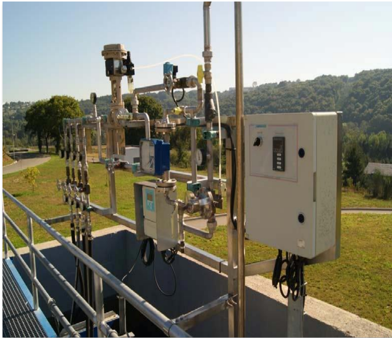
Inline pH control system with pH electrode
