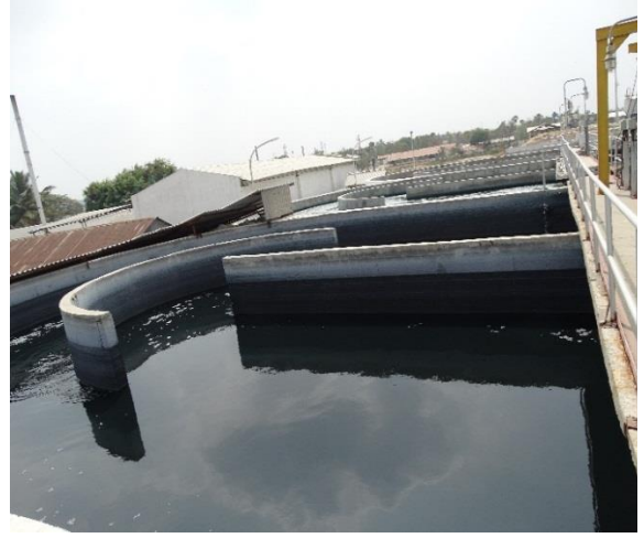
Storage and Homogenisation Tank
