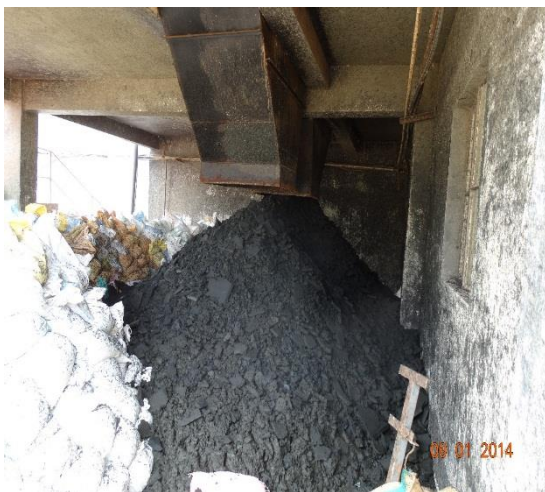
Sludge Dewatering System
